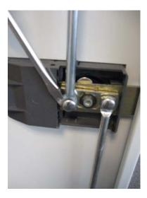
2) While holding the door and pressing firmly to push the lock out of the door, use a screw driver to press down the plastic tabs found on the top and underside for the lock. When this is done firmly press the tab on the back of the lock to disengage the lock from the door.
