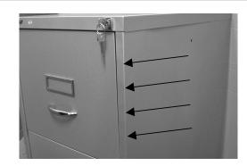
If there is a dent anywhere from top to the bottom of the right side panel, near the front corner, this may also affect the function of the locking bar.
