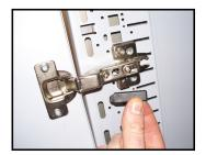
Open the cupboard door, you will see the hinges attached to the carcass with a small black plastic cover. You will need to remove the cover to make adjustments
