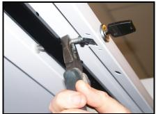
Using a pair of pliers clasp the bar of the lock
