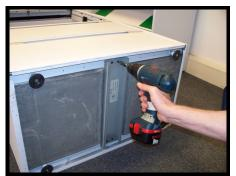
Fix into place by attaching the holding plate with the 4 screws provided.
