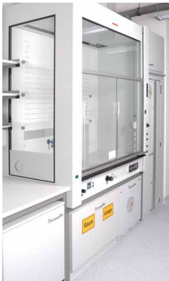
Fume hood with volume flow control. The special underbench cabinets to store acids and alkalis and the separate FW 90 hazardous materials cabinet have a separate extraction system.
